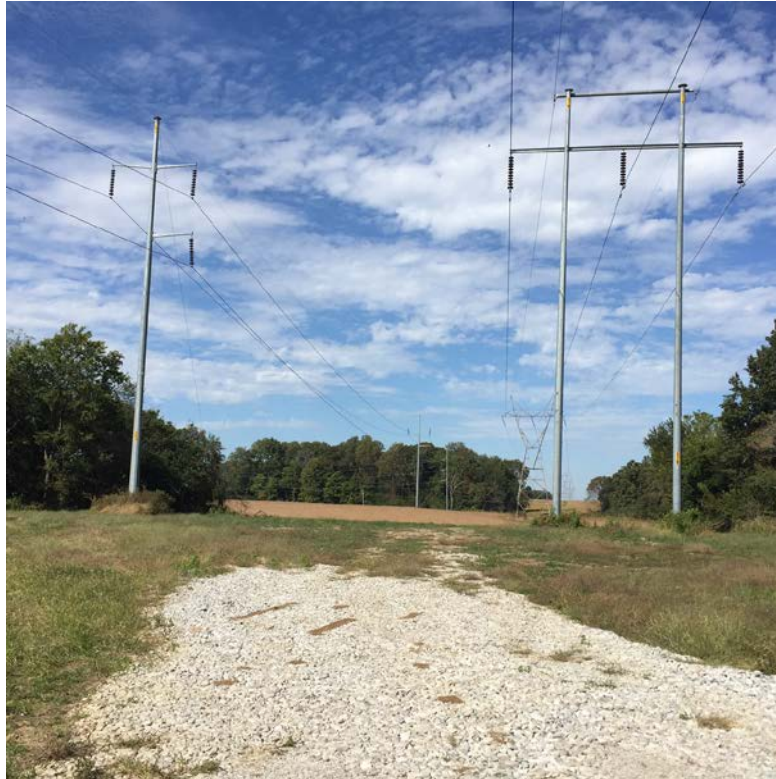
Figure 4 Overhead electric transmission lines crossing KY 115
